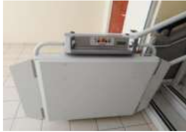
Wheelchair lift for the disabled, where needed – interior spaces
