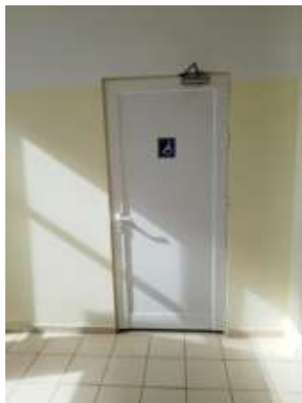
Toilets for the disabled in every building
